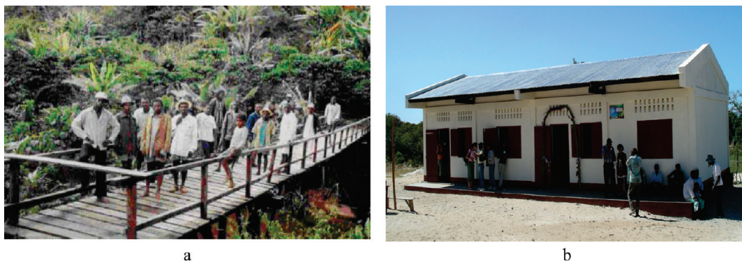
Figure 11. (a) Sarondroina bridge in Zahamena, Madagascar. (b) Primary school in Ambodivahibe, Madagascar. (Photographs by (a) Mamitiana Rakotozafy and (b) David Kingston).
